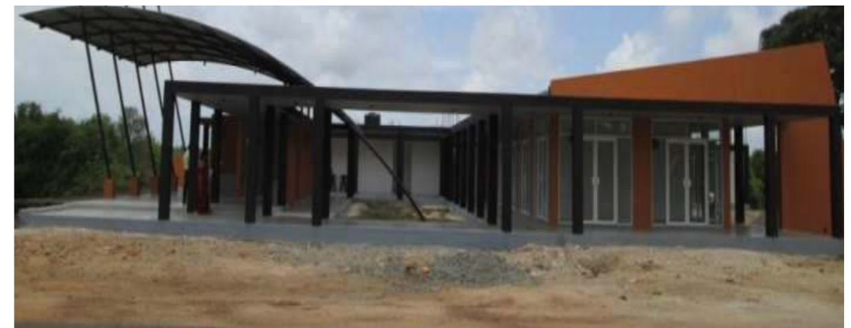
Madurankuliya Comfort Centre
